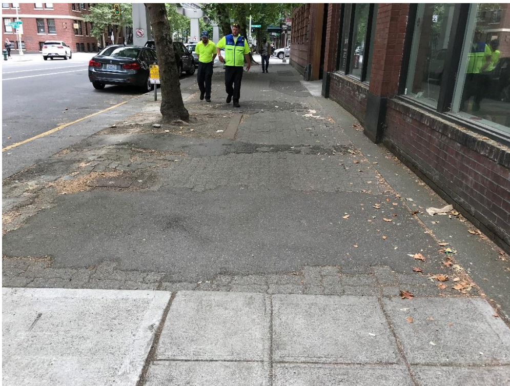
Figure 4: View south from roughly 120 ft north of Blanchard St.
