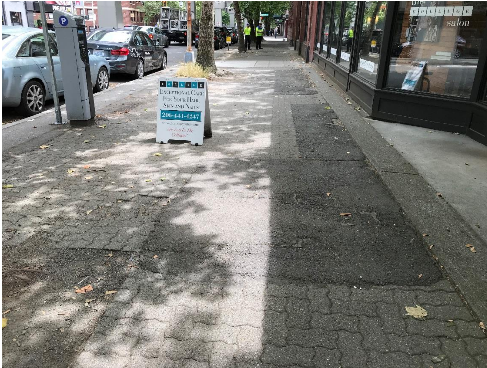
Figure 5: View south from roughly 225 ft north of Blanchard St.
