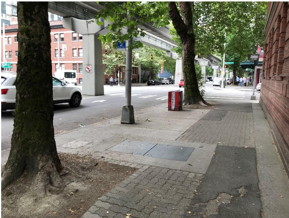
Figure 2: View south towards the corner of 5 th Avenue and Blanchard St next to the SPU vault.
