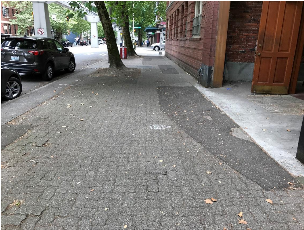
Figure 3: View south from roughly 80 ft north of Blanchard St.
